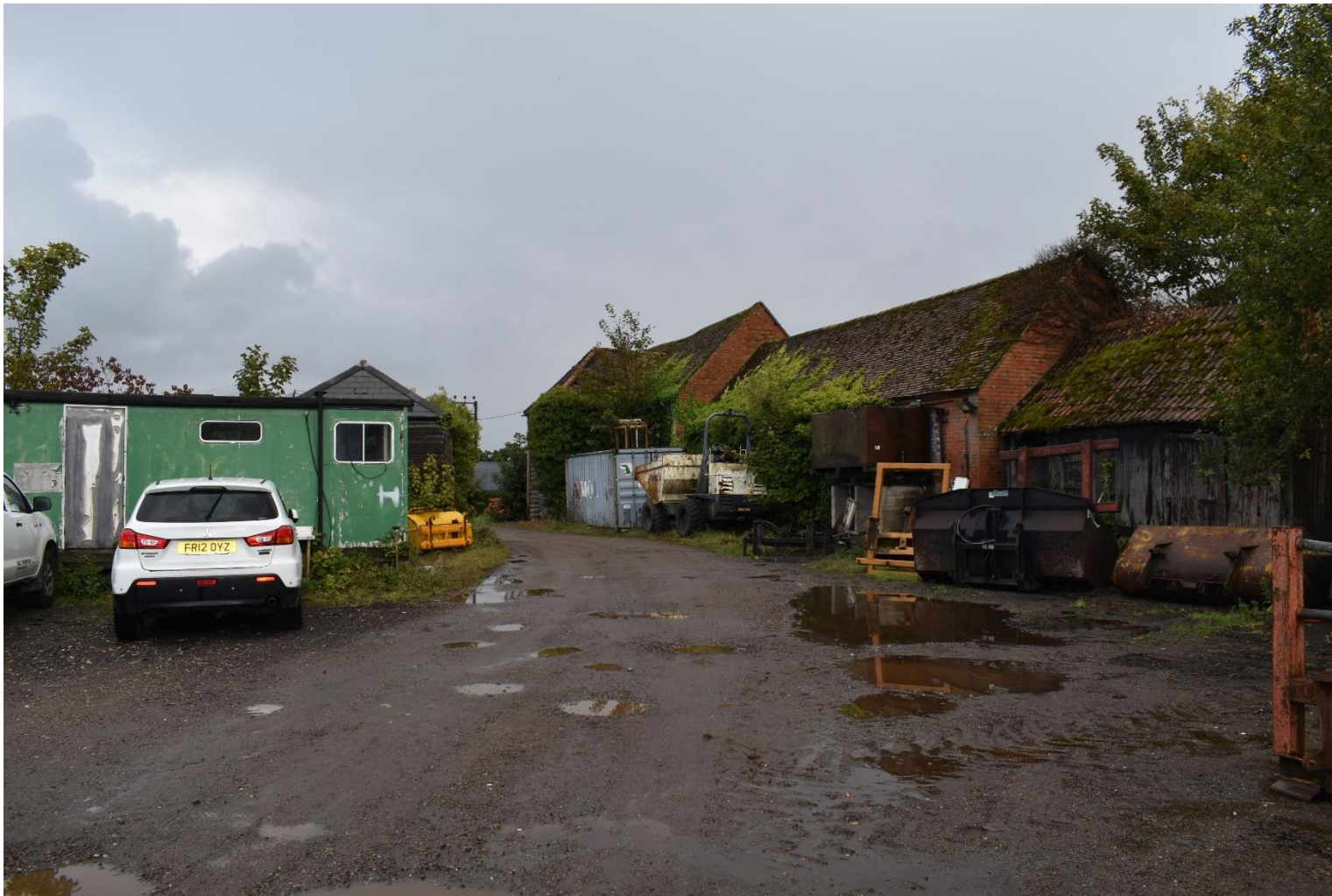
Plate 18: View across the yard towards the rear of the listed building of the original yard (facing ESE).
