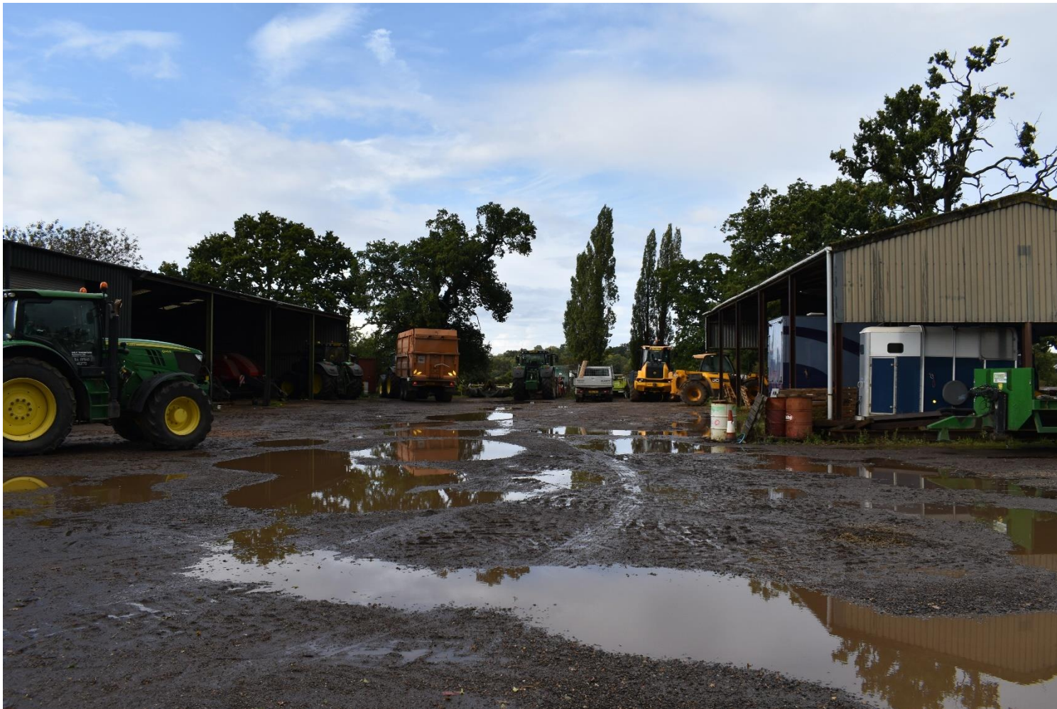
Plate 20: View across the yard (facing N).
