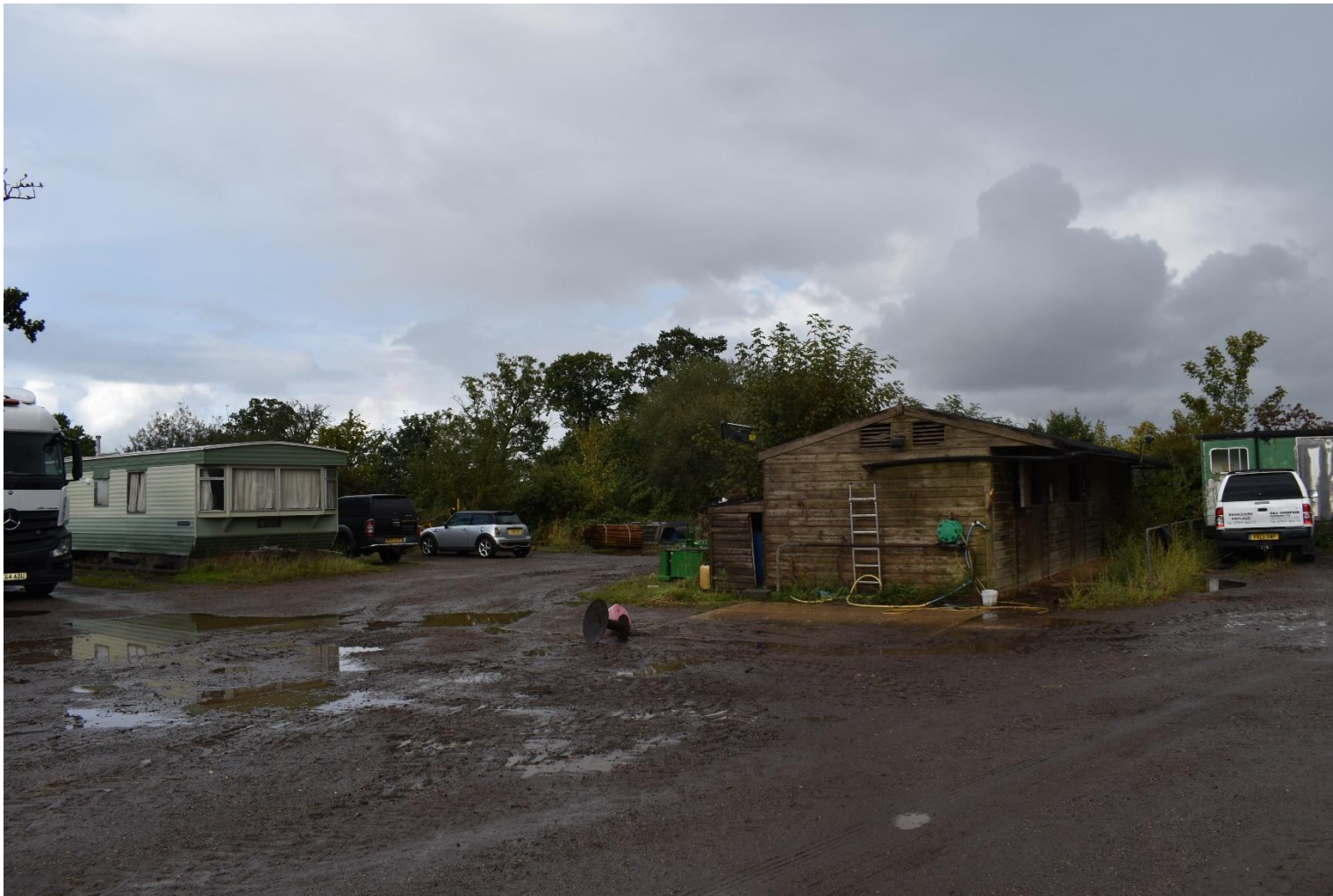
Plate 19: View across the yard (facing NE).
